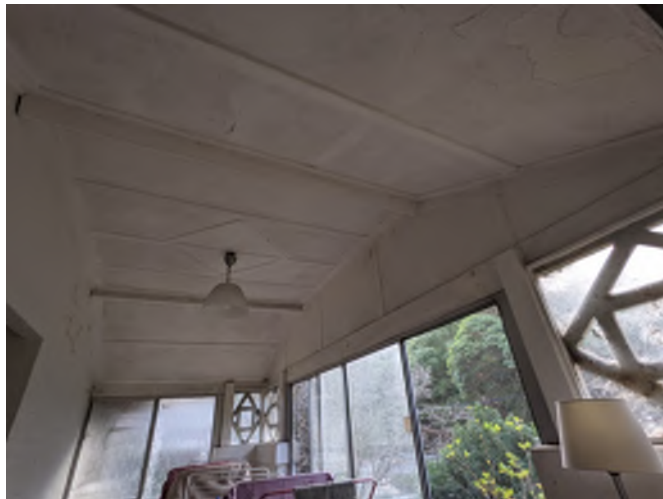
Photograph 5: FCS walls, ceiling and gable of 19 Canberra Avenue (29/6/2021).
